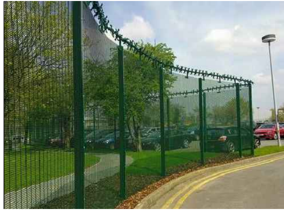
10' PERMEABLE FENCE, DESIGNED TO ALLOW VISIBILITY FROM THE OUTSIDE TO THE INSIDE WITHOUT COMPROMISING SECURITY
